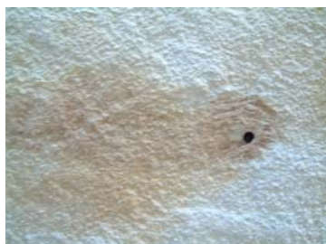
Figure 7. [a] External staining of harling
