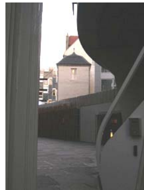
[b] New roof to pavilion tower
