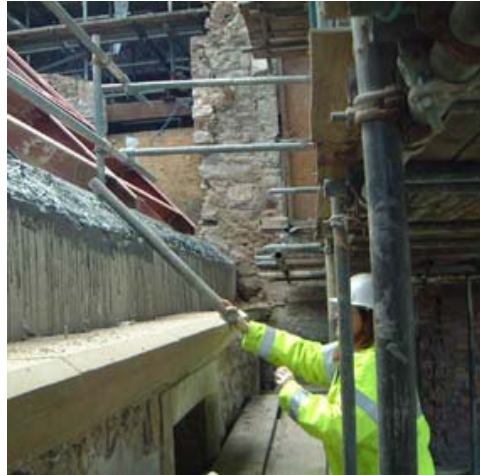
Figure 2. Building fabric at the start of the works
