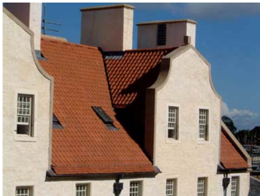
Figure 6. [a] New roof to South
