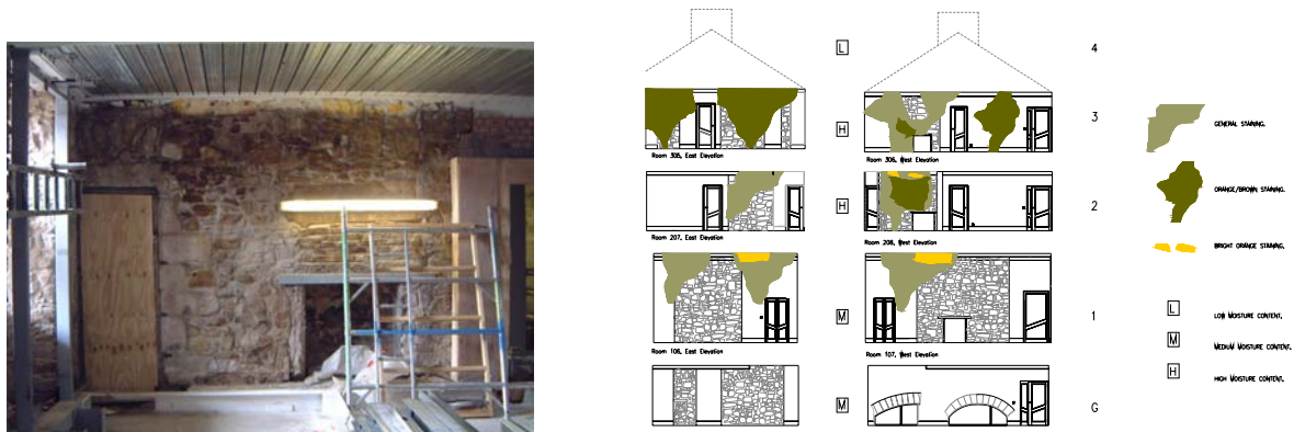
Figure 8. [a] Internal wall and fireplace showing staining- Stone discolouration [b] Mapping of staining
