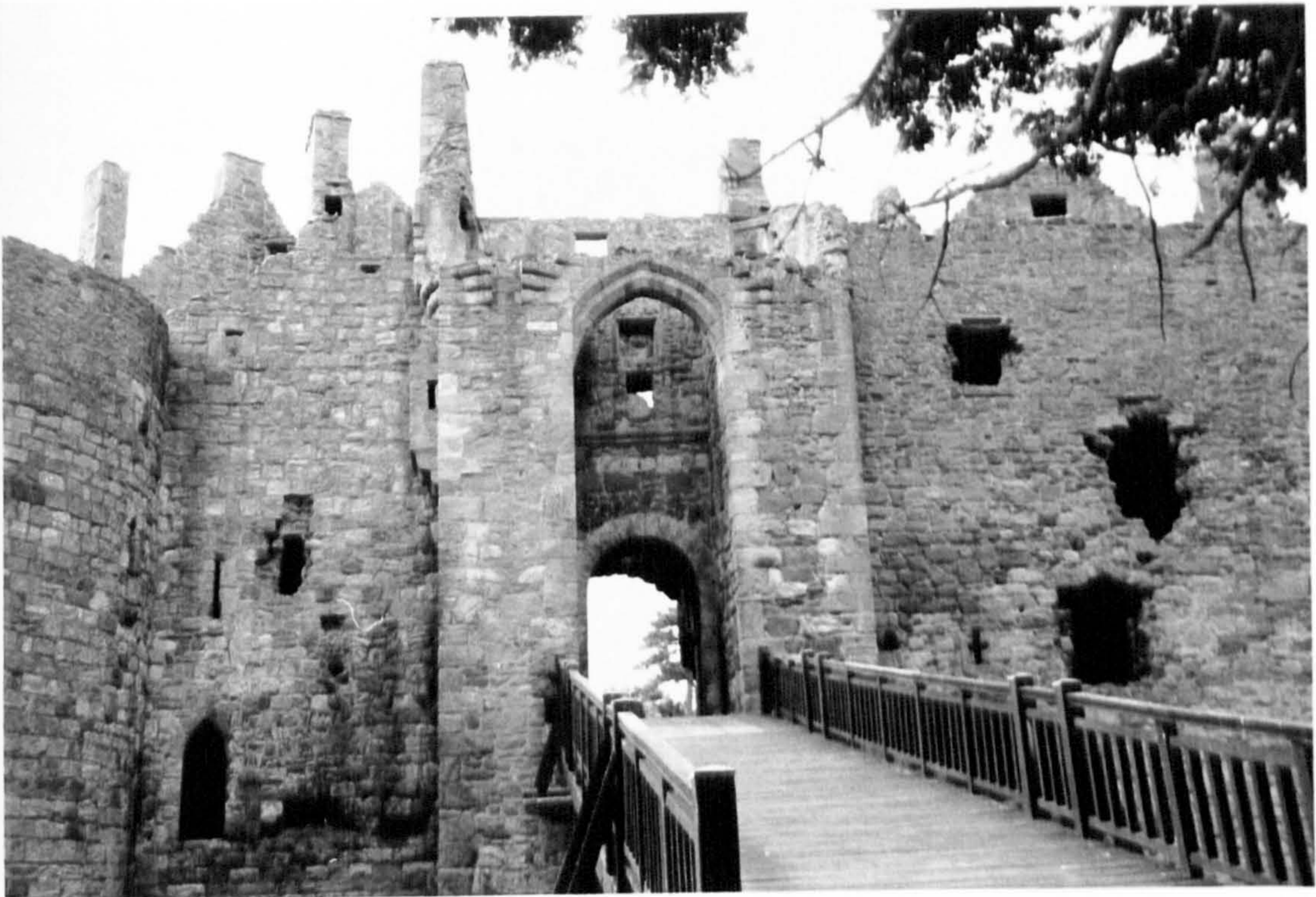
Plate 2. 13th century postern and 15th century gatehouse. Dirleton, from the west.
