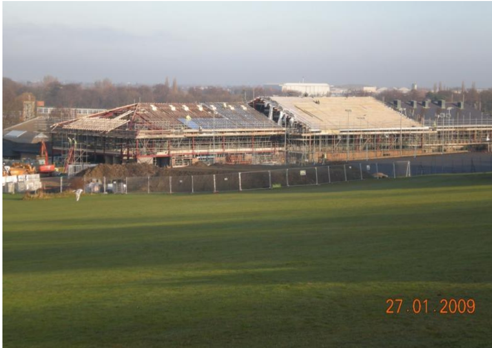
Photo 5.2 The new building being constructed on the large South site
