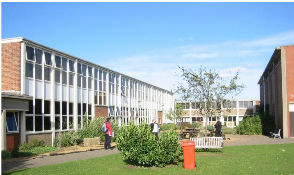
Photo 6.1 Existing buildings at St Augustine
