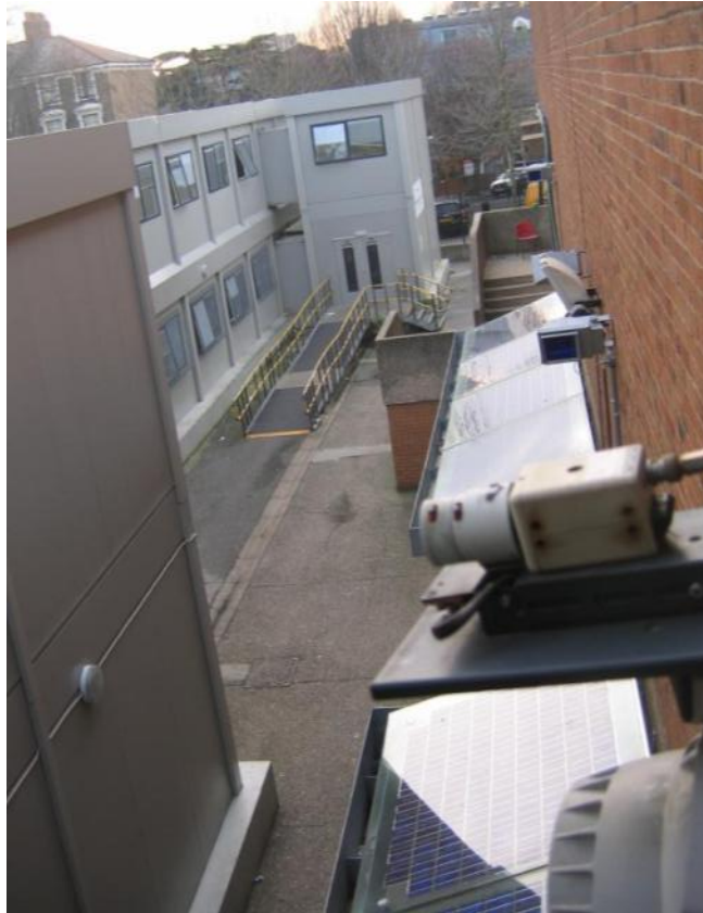
Photo 5.8 A small area of PV panels acting as sun screens for windows below. The photo also demonstrates the cramped site in a built up area, suggesting that biomass is an unsuitable choice due to its space requirements for storage and delivery of fuel
