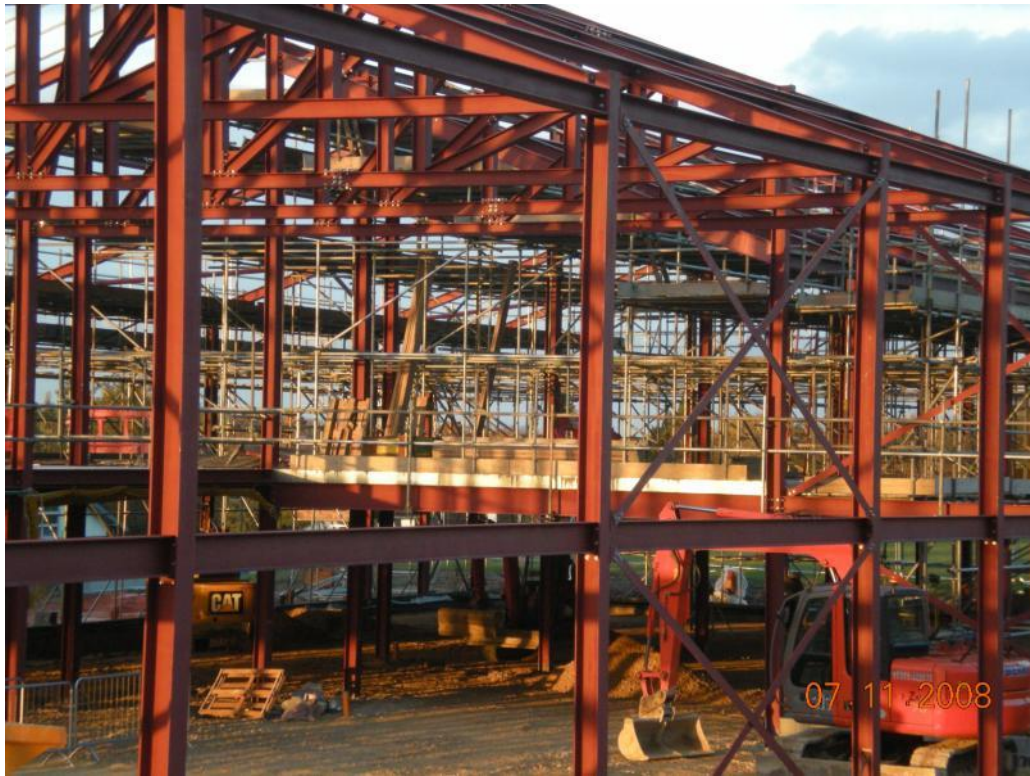
Photo 5.4 The steel frame of the new teaching block being erected in 2008
