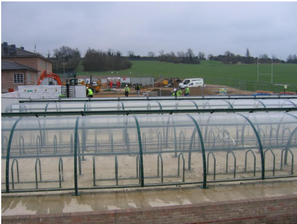
Photo 5.3 640 new bike racks, allowing parking for 1280 bikes, being installed – this is by far the most common mode of transport for pupils
