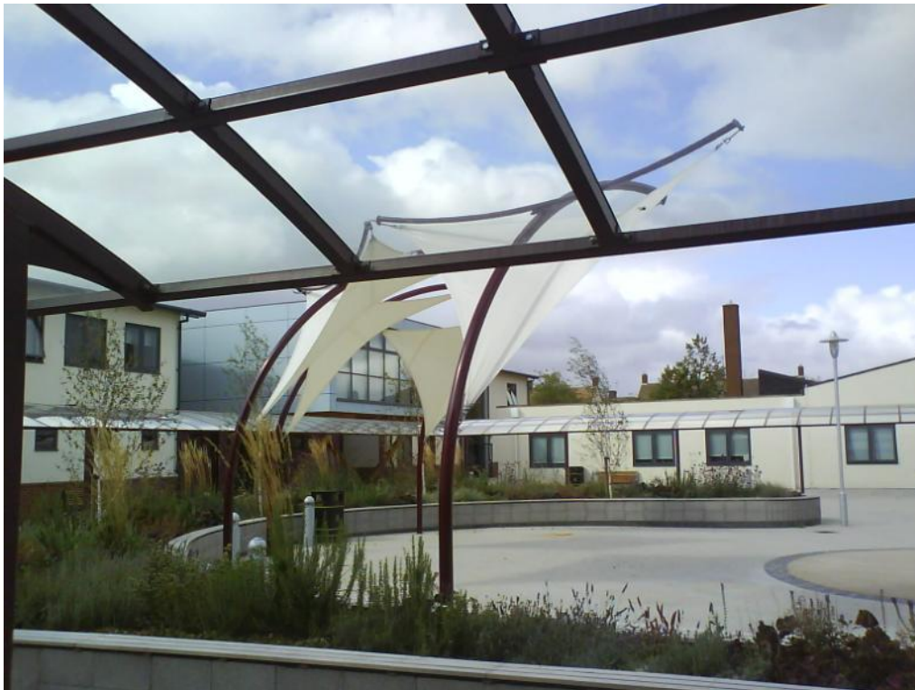
Photo 6.5 The finished courtyard linking new and refurbished buildings at St Augustine. Behaviour and academic results at the school have improved since the project.
