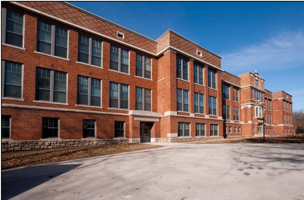
Figure 5. Renovated Bancroft School Building. Source: Thebancroftschool.com, 2016.
