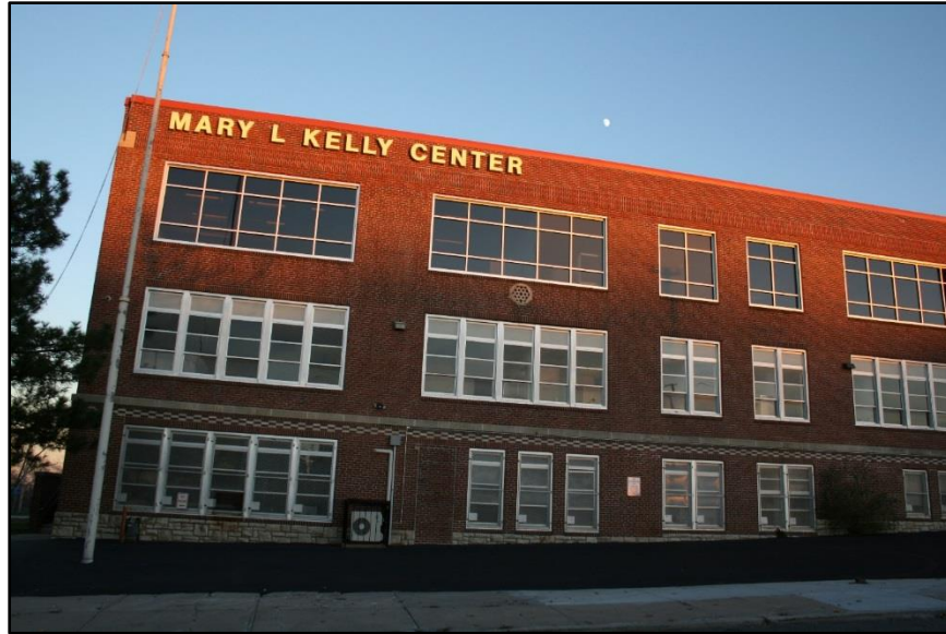
Figure 6. Exterior of the Mary L. Kelly Community Center. Source: KCtechschool.com, 2016.
