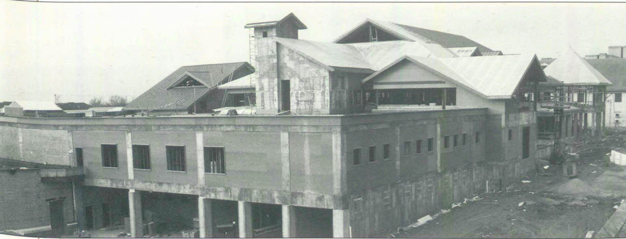
Clydesdale Hall under construction.
