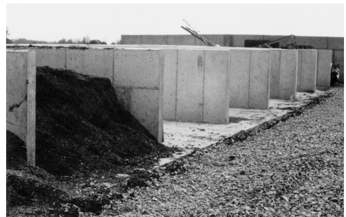
Figure 2. This unroofed composter with concrete bin walls serves a large finishing operation.
