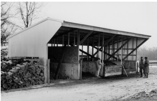
Figure 1. This roofed composter has concrete bin walls with a roof overhang to protect the work area.
