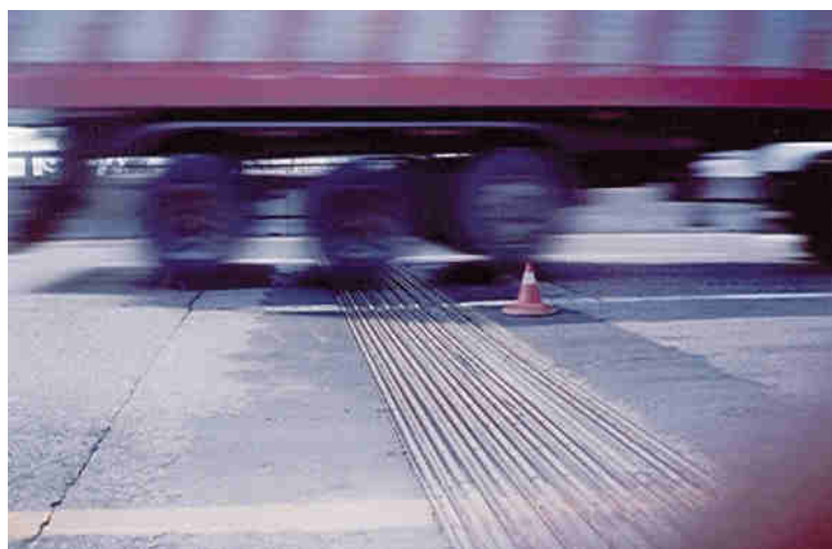
Figure 3. Loss of tire/pavement contact during the passage on the BEJ.
