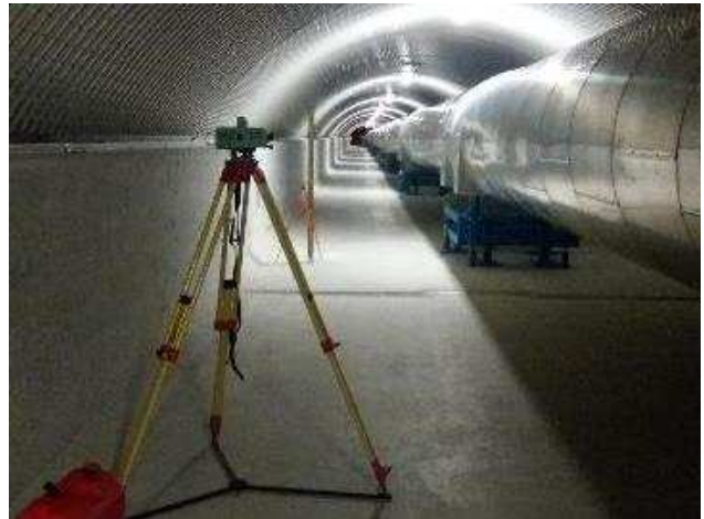
Figure 4: DNA03 station in the Tunnel.
