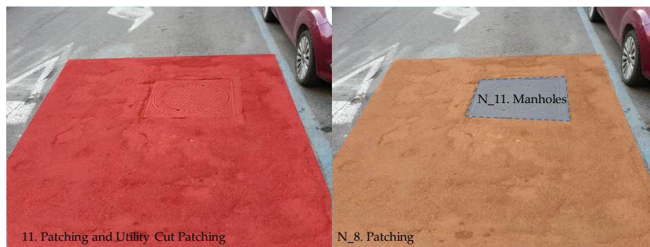
Figure 8. Example of manhole distress identification guidelines.
