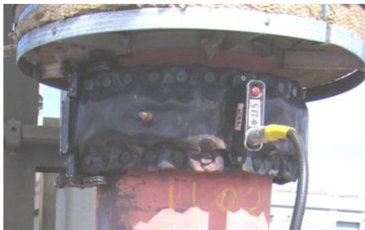
Figure 7.4: Picture of inflatable transducer ring used to perform guided wave inspections at Port of Liverpool power station.
