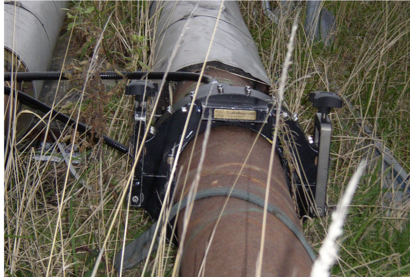
Figure 7.9: Ring of transducers in use for guided wave inspection.
