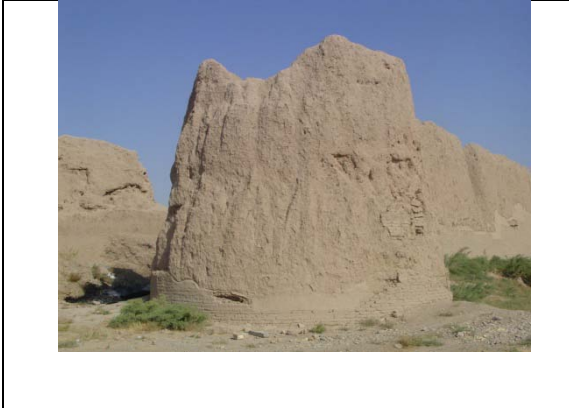
Fig. 3.30 - Tūs – a mudbrick bastion at the Merv gate of the outer city walls.
