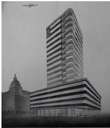
Fig. 3 Skyscraper with a welded steel frame (Bollettino Tecnico Savigliano 1934).
