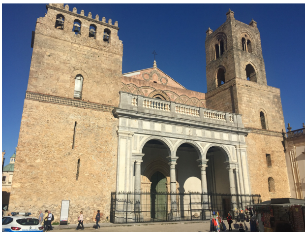
Figure 2. Main façade of Cathedral of Monreale
