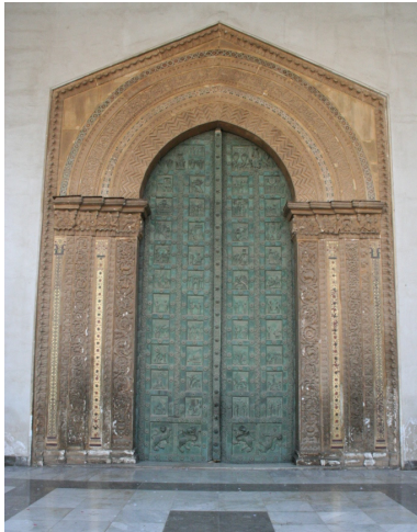
Figure 4. The main portal of the Cathedral of Monreale before the restoration
