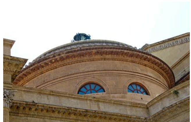
Figure 4. View of the exterior of the dome
