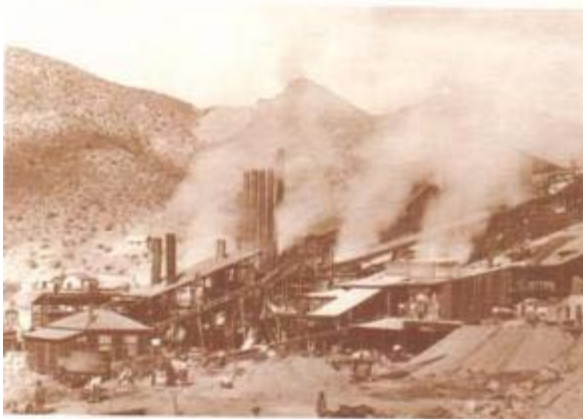
The Detroit Copper Company smelter in 1896. This site is now under a mine dump on the south side of the Morenci pit.
