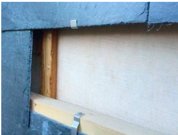
Fig. 2. (a) The MgO-board is placed facing the air gap, which is behind the siding boards made of natural slates; (b) Salty water drops on a vertical MgO-board on the side that faces the insulation filled cavity inside the wall.
