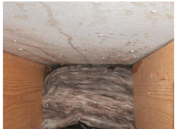
Fig. 2. (a) The MgO-board is placed facing the air gap, which is behind the siding boards made of natural slates; (b) Salty water drops on a vertical MgO-board on the side that faces the insulation filled cavity inside the wall.
