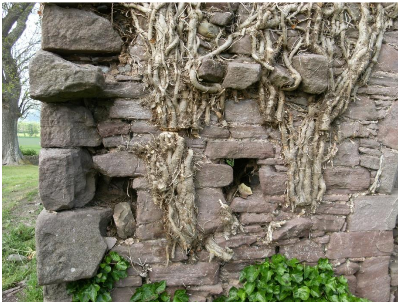
Fig. 5: The east gable of the church contains a large central pointed arch of dressed stone within a Junction between random rubble and external squared rubble on east gable, showing differences between block sizes and bed heights.
