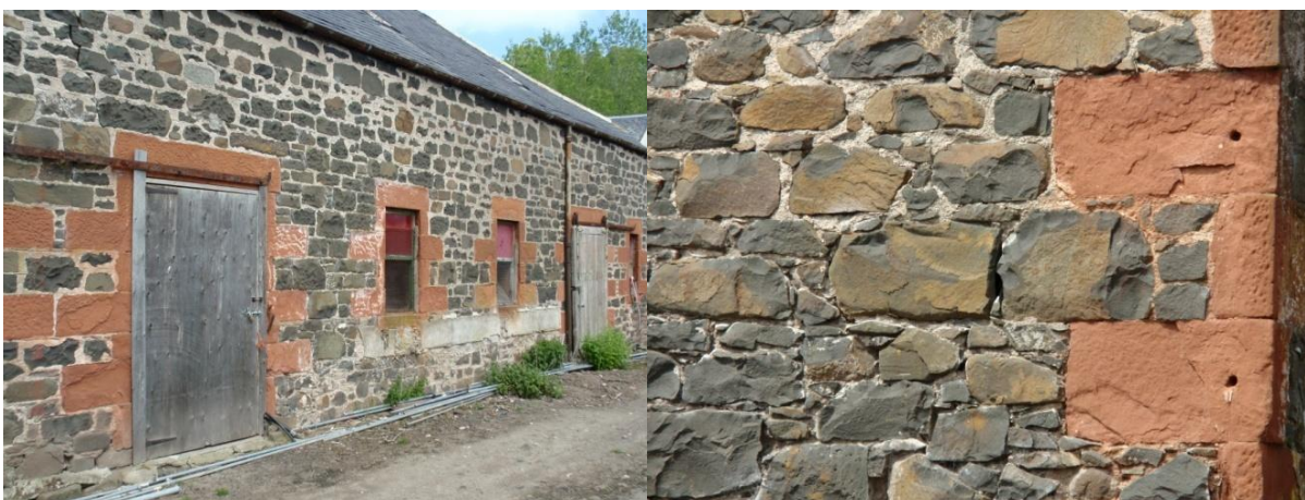
Fig. 18: Farm steading just outside of Rait built with locally sourced random rubble whinstone walling and fine grained, orange/red sandstone dressings. The red sandstone would have been sourced from the Ballindean area for its larger block sizes and brought in for door and window surrounds.
