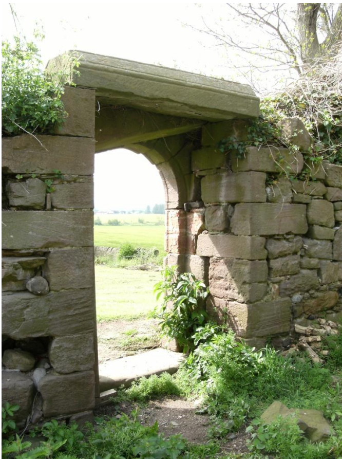
Fig. 11: Entrance to south wall, showing lintel made from reused grave slab.
