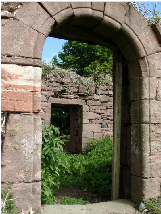
Fig. 4: The two entrances to the building; round headed, roll-moulded archway of south entrance and square headed north entrance.
