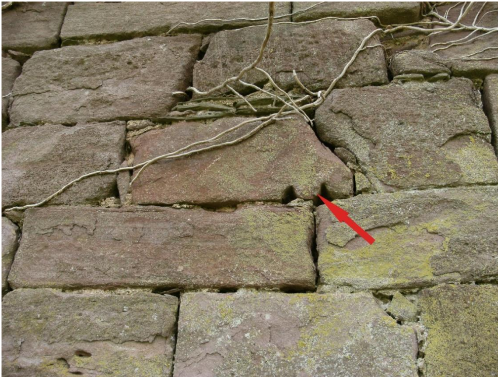
Fig. 10: Reused masonry block with moulded detail (arrowed) on west gable interior.
