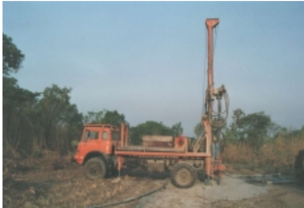
Plate12. Project drilling rig at BGS18
