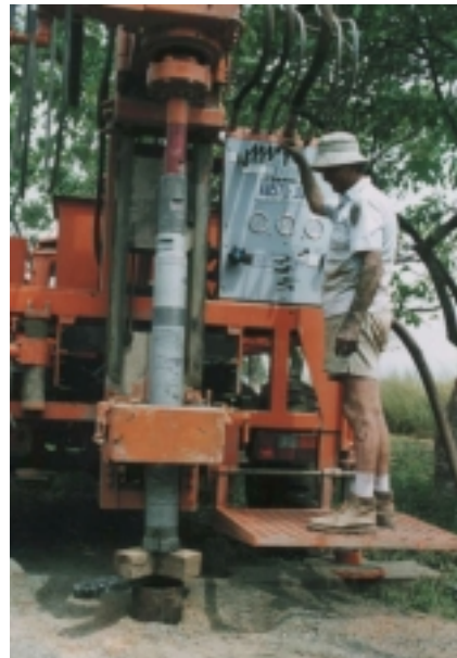
Plate 15. Down the hole hammer used for hard rocks
