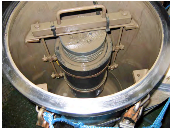
Before cleaning photograph showing the high levels of sediment contamination experienced in 2007
