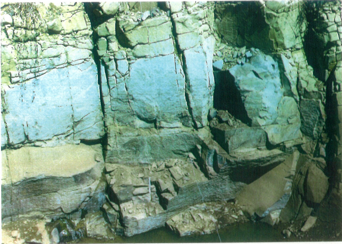
Photograph 2.1a Example of the compact lower layer of a lava sequence showing sub-vertical jointing
