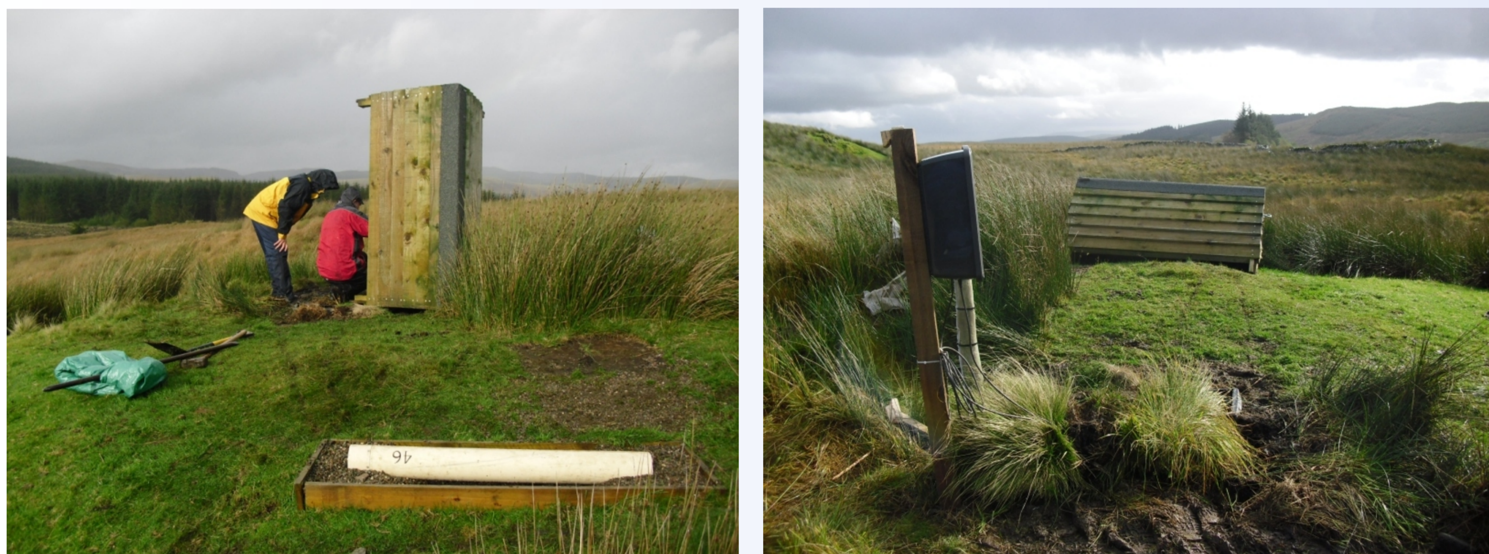
Figure 1: Installation of Channel 1 (North) induction coil at Eskdalemuir [55.314° N, 356.794° E] in the Scottish Borders, UK. Left image: The coils (white tube, foreground) are located in a rural valley (background), protected from wind, rain and snow under a non-magnetic wooden cover (shown upright in midground). Right image: Looking eastward to the enclosed coil under wooden cover. The signal is digitized close to the coil before being converted to a higher voltage at a breakout box (mounted on the post) and sent to a logging computer in a vault approximately 150m away not shown).
