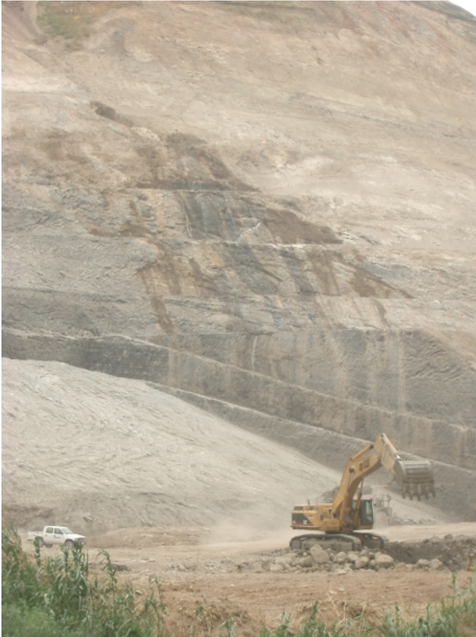
Figure 1.7 The Eastern Springs site, Maqarin (northern Jordan) in June 2004 after dam construction began. At the top left of the image is the remains of the tunnel (Adit A-6, Figure 1.6b) which hosted several of the seeps of the Eastern Springs. The hyperalkaline waters can be seen flowing down the excavated rock steps towards the valley floor.
