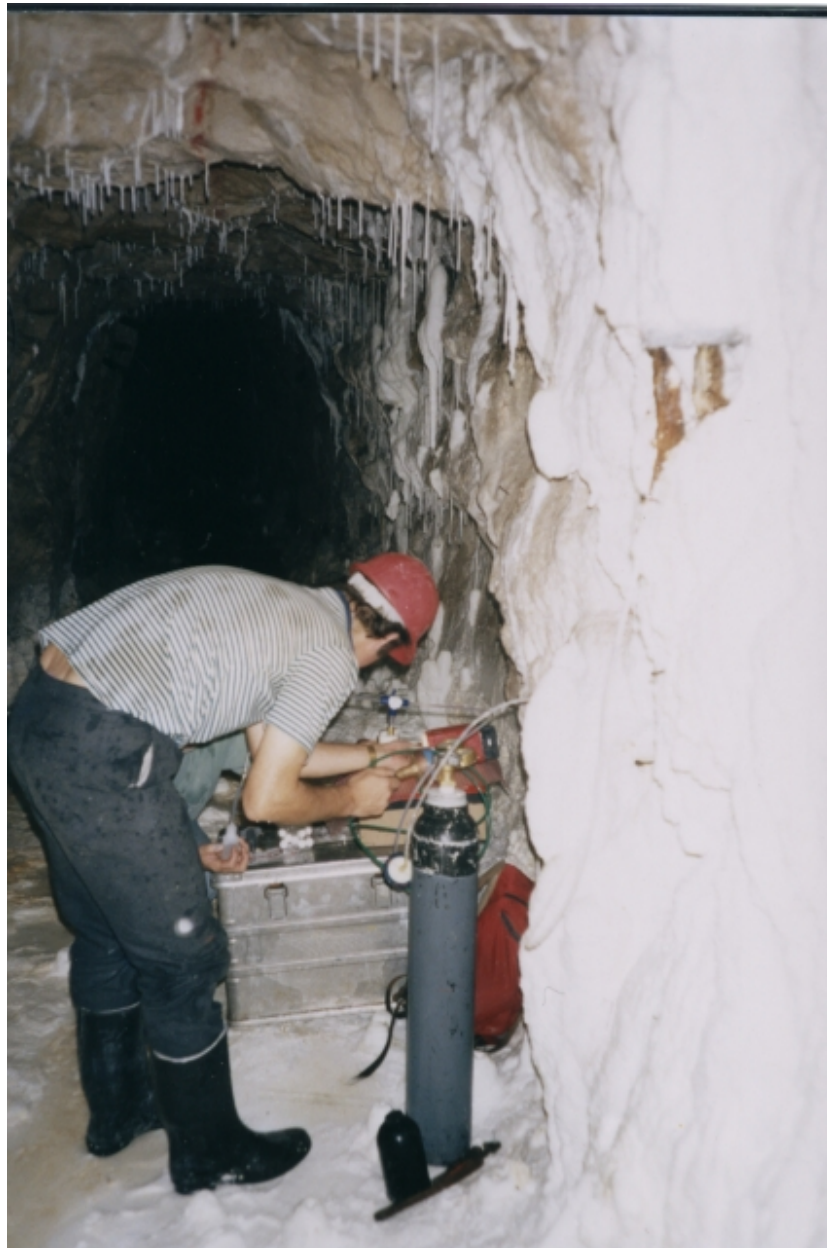
Figure 4.42 View of Adit A-6 showing typical thick carbonate travertine precipitates on the tunnel wall (consists of calcite, aragonite vaterite and minor CSH (Milodowski et al., 1998a))
