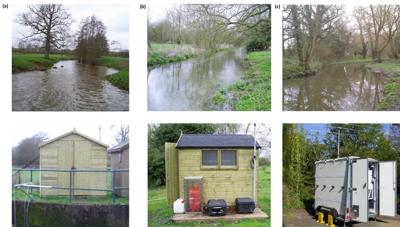
Fig. 3. Photographs of the river monitoring stations. River systems (top row – taken in March 2010): (a) River Enborne at Brimpton (Great Britain National Grid Reference, SU56776477), (b) River Kennet at Clatford (SU16016885) and (c) The Cut at Bracknell (SU85837050). Monitoring stations (bottom row – taken in April 2010): (a) River Enborne at Brimpton (SU56776477), (b) River Kennet at Clatford (SU16016885) and (c) The Cut at Bray (SU91397866).
