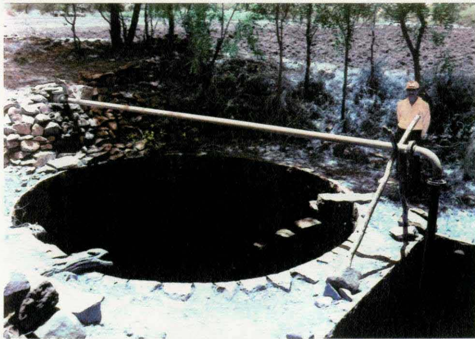
Figure 2.2 Dug well lined at the surface with basalt blocks.
