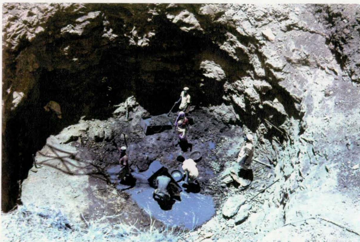
Figure 2.4 The deepening of a large diameter dug well.
