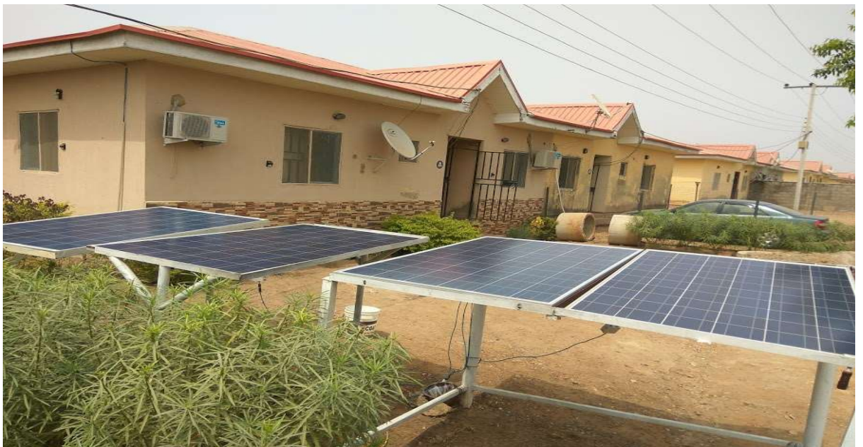
Figure 66. Solar array installations at Kuje estate Abuja
