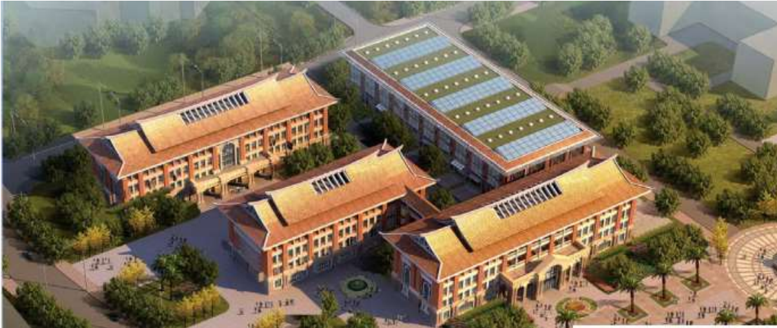
Figure 136. Campus building at Xiamen University, China, showing the roof top installation of 150 kW PV array for DC micro – grid [13].
