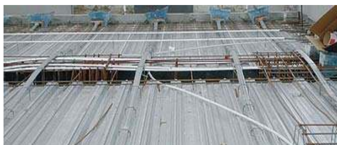
(b) Decking prior to placing concrete
