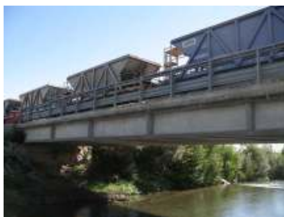
Figure 5 "Terdoppio" bridge under final testing
