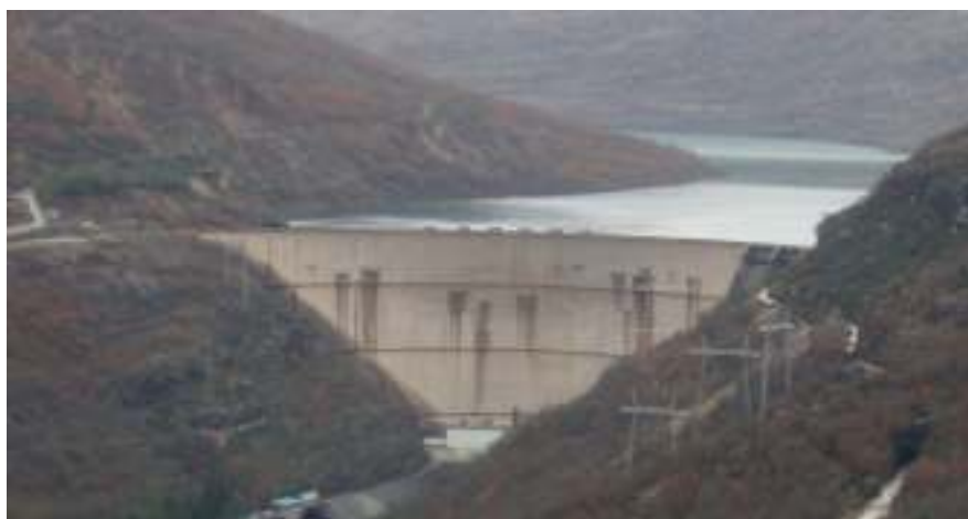
Figure 2 Grančarevo Arch Dam - photograph
