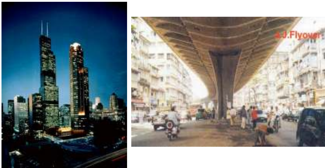
Figure 4 311 South Wacker Drive, Chicago (to the right of the Willis Tower) and The JJ Hospital Flyover in Mumbai. Both made significant savings through the use of high strength concrete.
