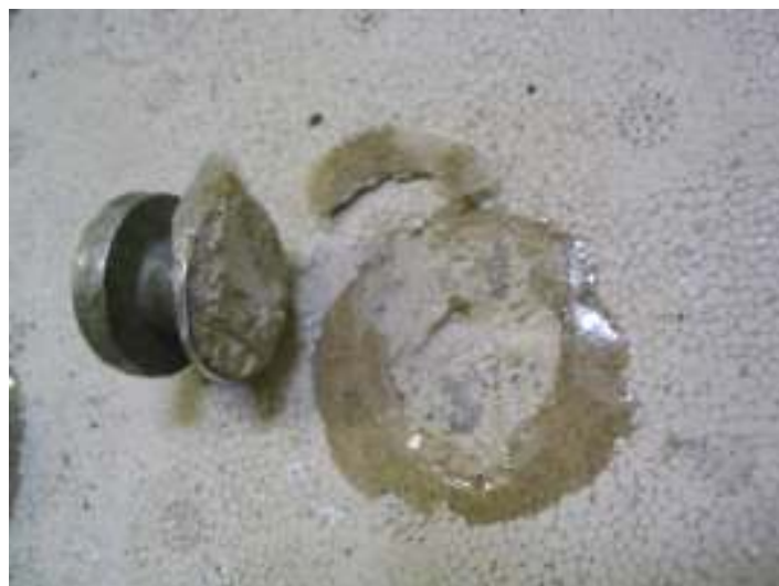
Figure 4 Cohesive failure of a joint (Pull-off test)
