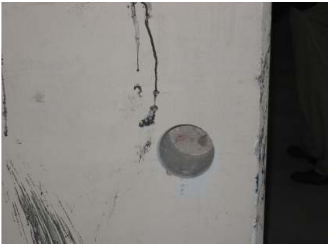
Figure 7 Core taken from a concrete column in Zone 3
