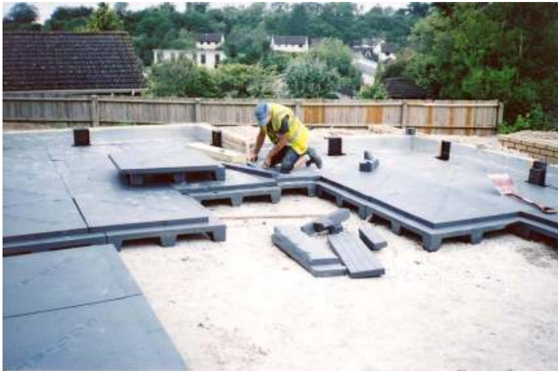
Figure 1 Placing the insulation units
