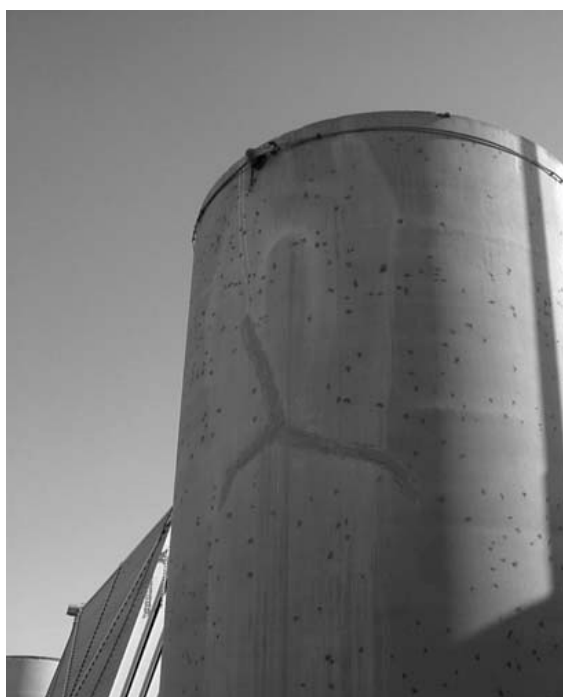
Figure 5 Thermal cracks
