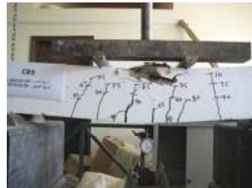
Figure 11 mode of failure CB5
