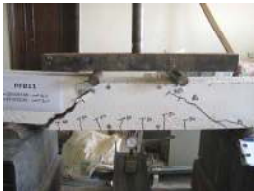
Figure 14 mode of failure PFB11
