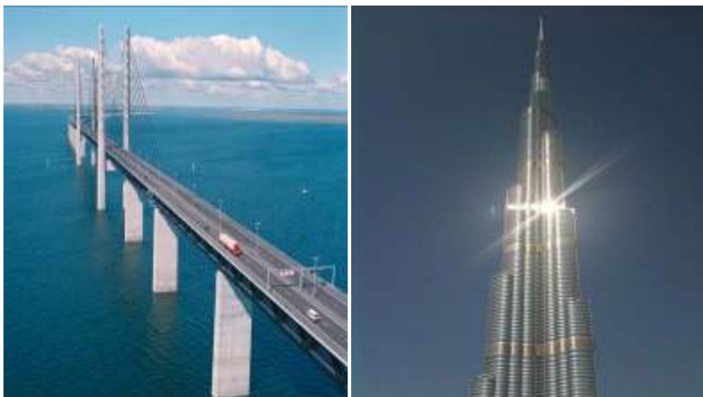
Figure 1 The Øresund link and Burj Khalifa – two projects that have used binary and ternary blend concretes for rheology and durability
