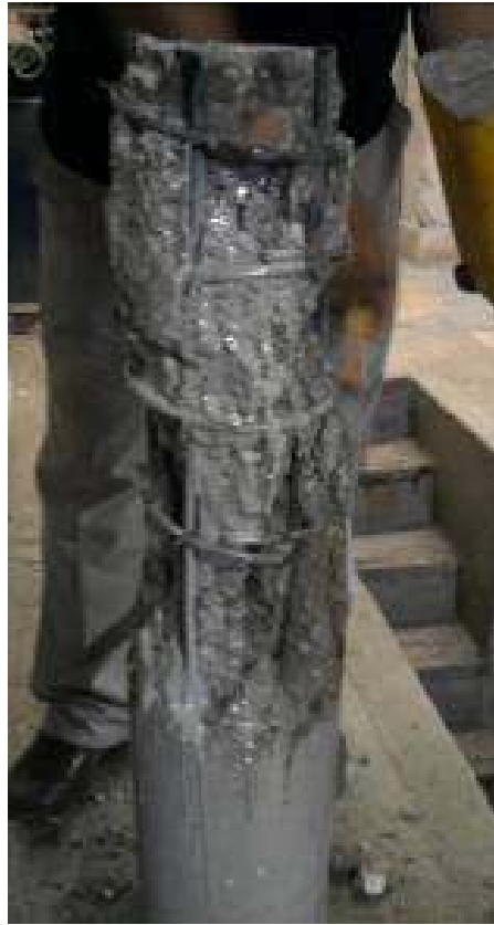
Figure 4 Repairing the top part of the loaded column (C3) before strengthening
