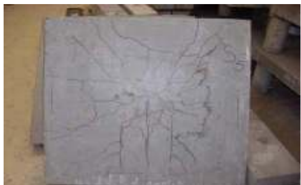
(e) Slab S5; HSCC with steel fibres (0.75%)
