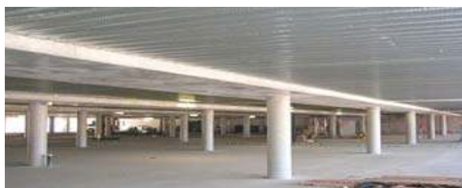
(a) Soffit of a one-way slab and beam floor system
