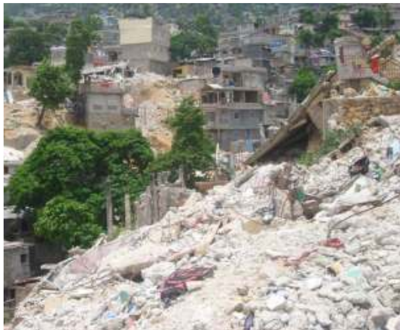
Figure 3 Photograph of a collapsed dwelling at Fort Mercredi, Port au Prince
