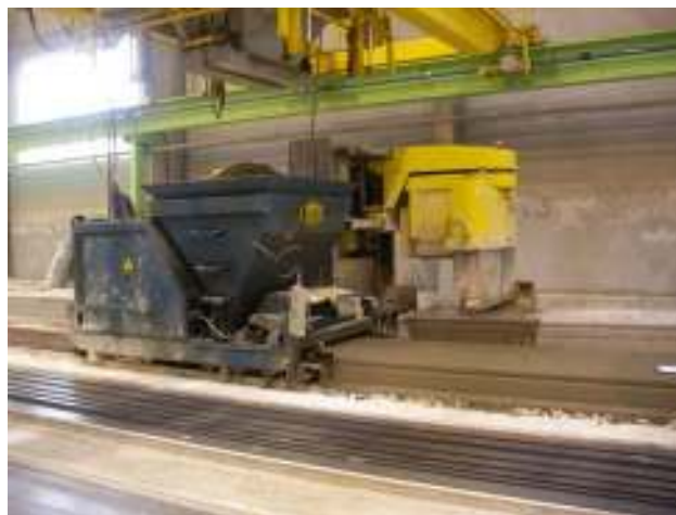
Figure 1 Moulding and sawing process of precast reinforced concrete floor slabs
