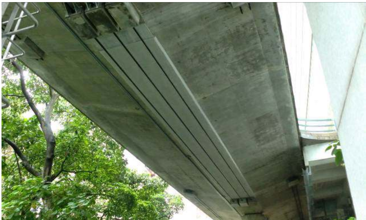
Figure 2 Bridge after strengthening works
