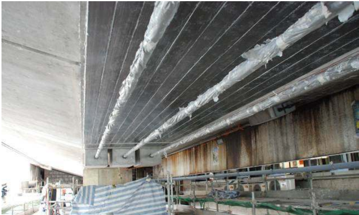
Figure 1 Prestressing bar and CFRP plate installation in progress
