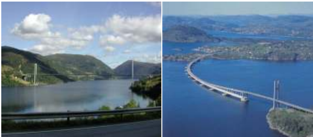
Figure 3 Kvisti Bridge has most of the central span cast in lightweight concrete, while the Norhordland Bridge floats across the fjord.
