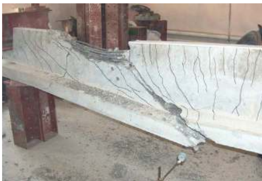
Figure 5 Breaking of beam F.P.04
