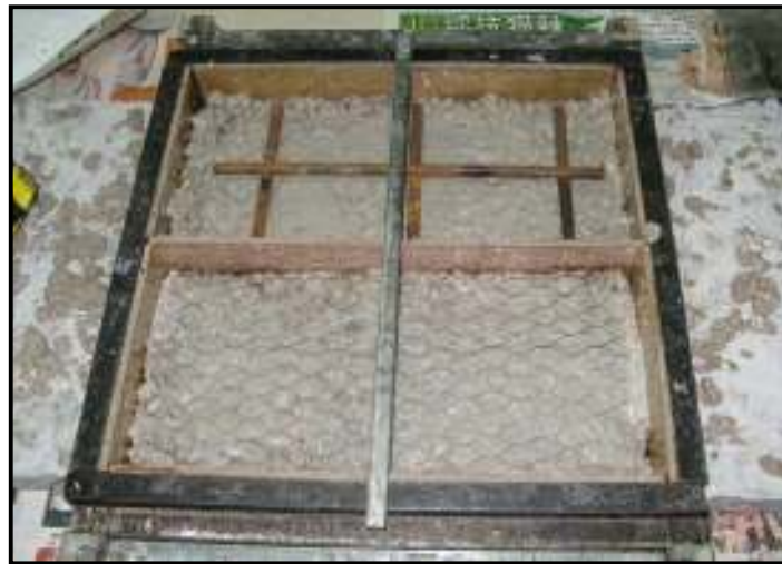
Figure 6 Casting of test specimen pair (top: with mesh reinforcement D503, bottom: with chicken wire mesh)
