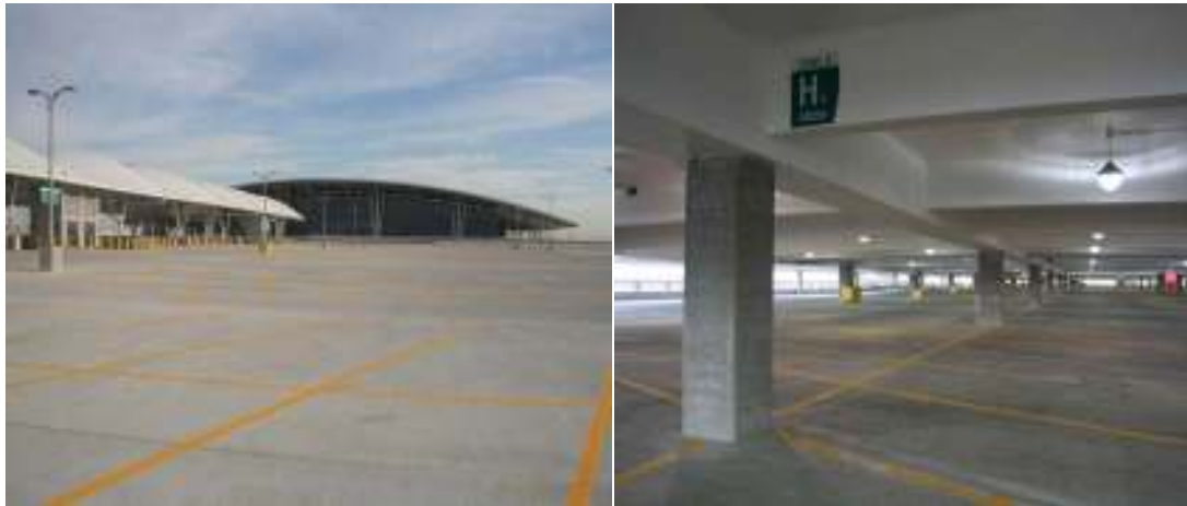
Figure 5 Indianapolis International Airport Parking Garage
