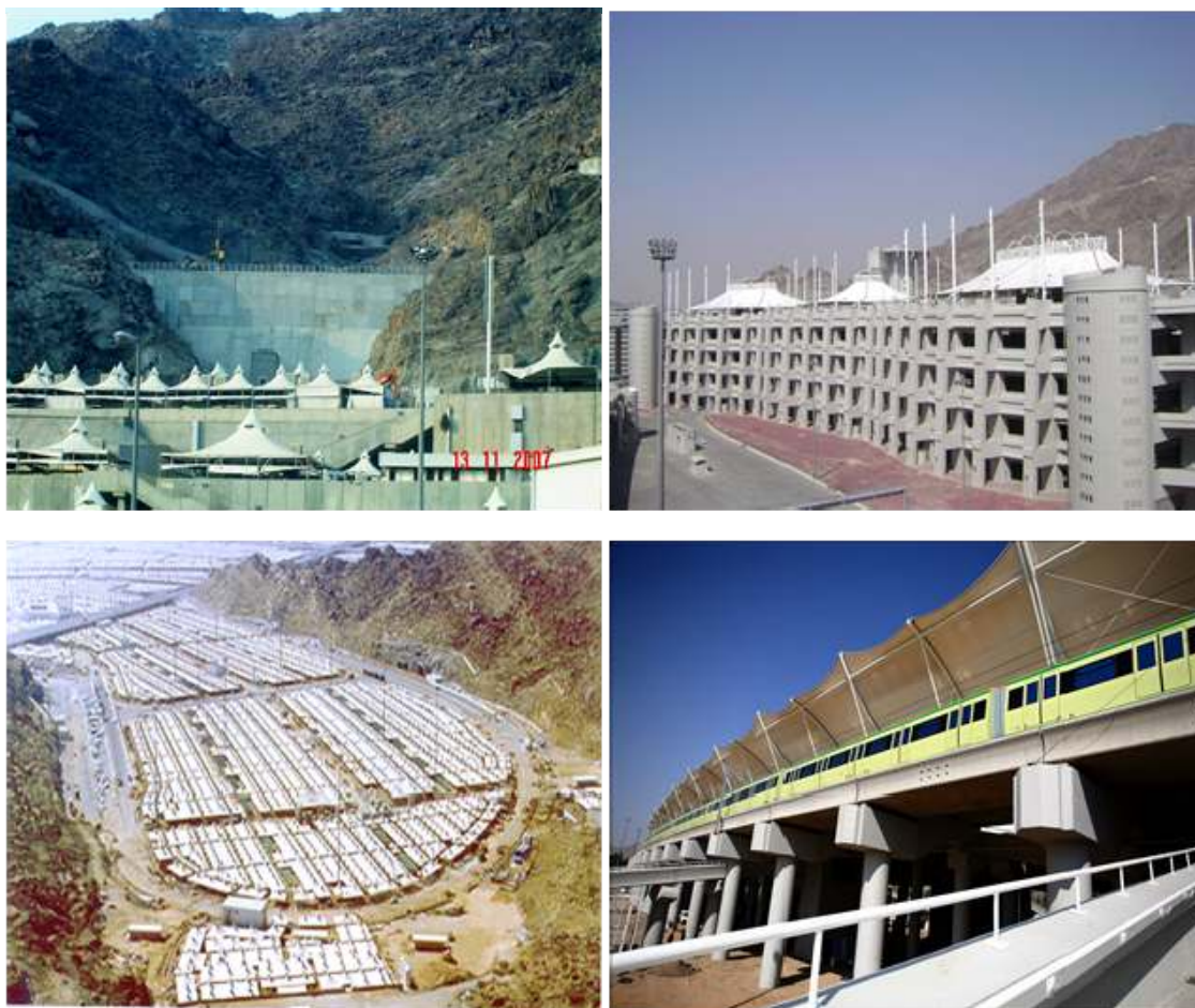
Figure 1 General Views of Four Mega Projects in Makkah AlMukarrama (Mecca) , KSA
