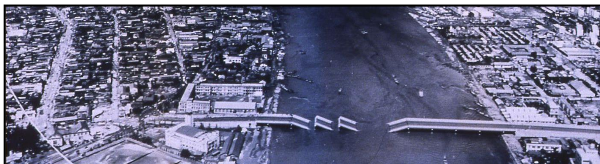
Figure 2: Showa Bridge collapse during 1964 Niigata Earthquake
