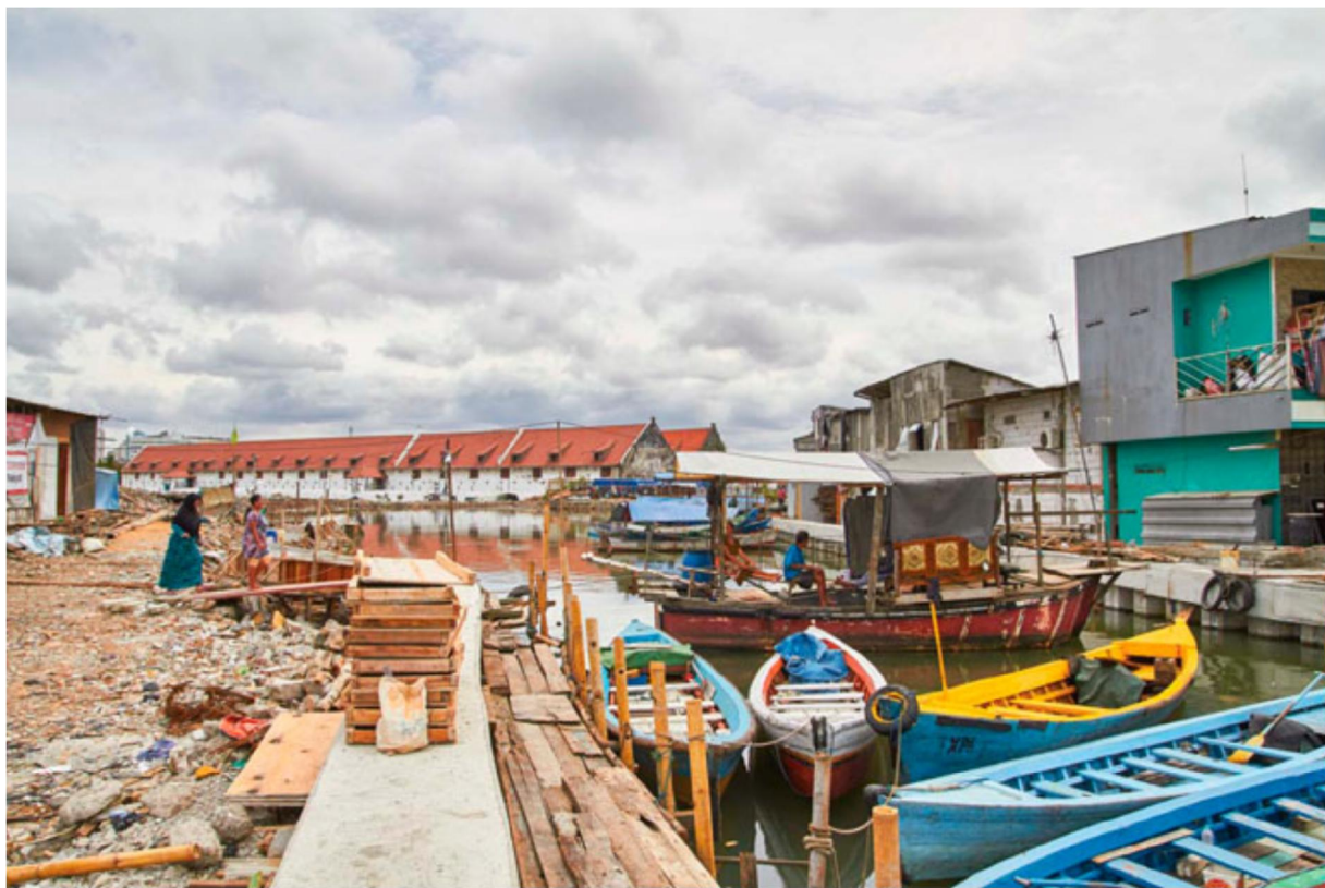
Figure 2. Preserved Dutch East India Company warehouses provide the backdrop to the ruins of the demolished neighborhood of Kampung Aquarium. Author’s photograph.
