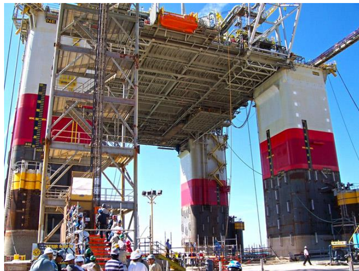
Figure 1.2 Photo of Blind-Faith, during topside construction: Courtesy of Aker Akaerner
