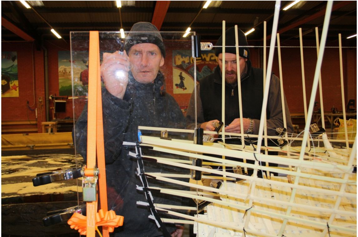
Figure 146. Dry-erase markers were used to draw on potential posts and planking termination points. These tentative lines were later reinforced by using steel flat stock clamped to the polycarbonate plates, providing firm anchor points for the ends of the ribbands. Newport Museums and Heritage Service.
