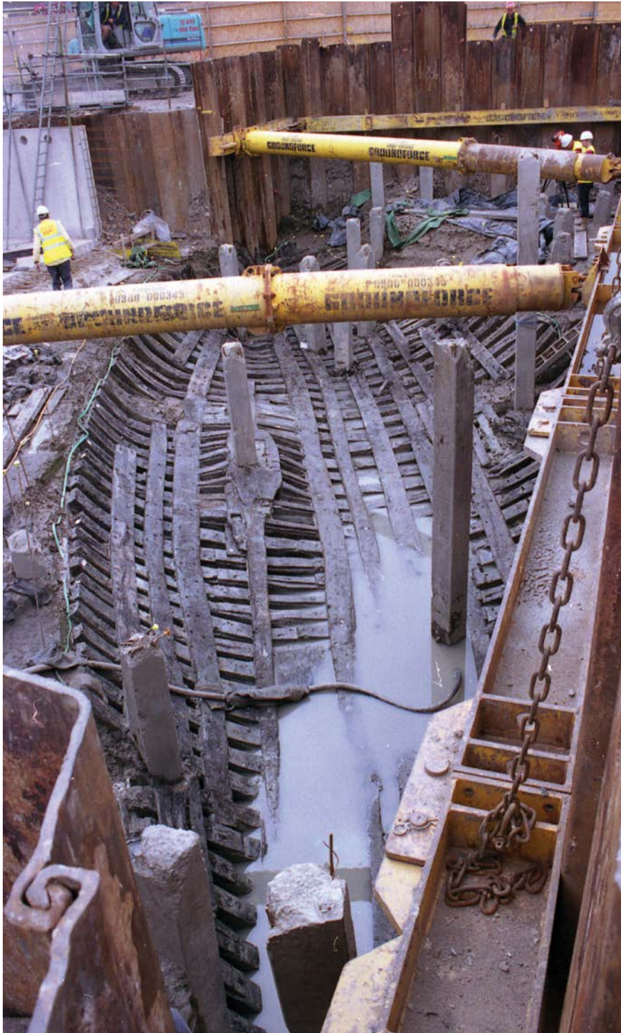
Figure 2. Excavated hull remains pierced by numerous concrete piles. Port side is to the left. Newport Museums and Heritage Service.
