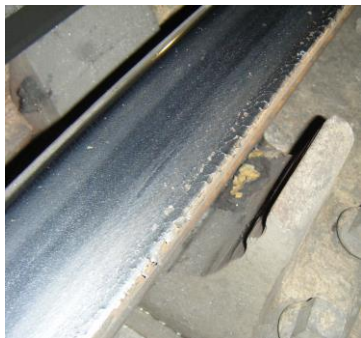
Figure 2: Example of a shelling defect observed on the LUL tracks
