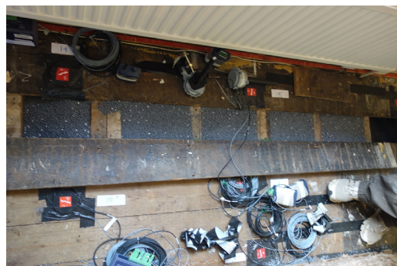
Fig. 2. The bead filled floor along the exposed perimeter wall.
