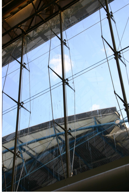
(b) London Waterloo Station, UK
