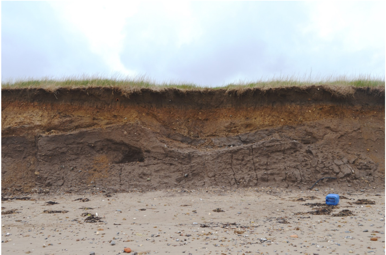
Figure 4.4. An example of a heavily-fractured till, east Yorkshire, showing vertical and horizontal joint sets.
