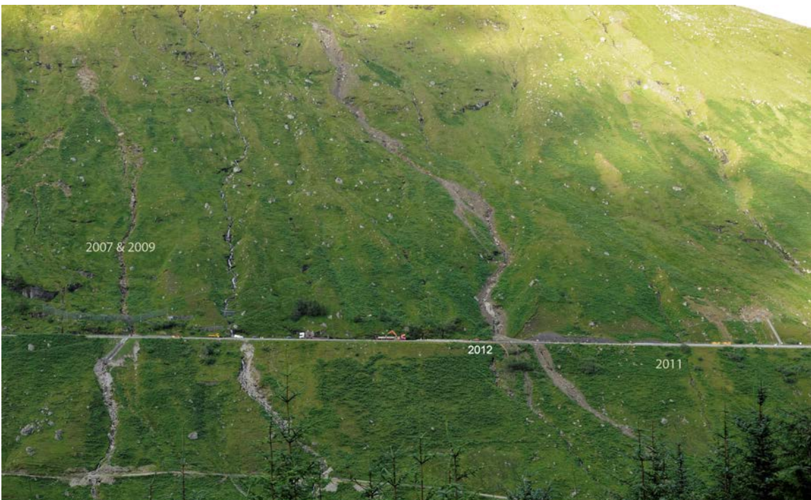
Figure 7 Recent debris flows on the A83 Rest and Be Thankful Pass
