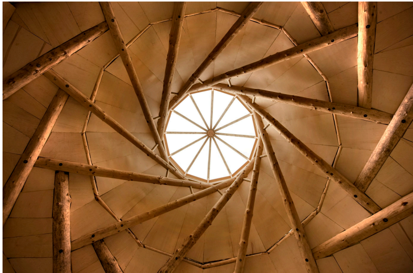
Figure 16. Roof light in the reciprocal roof of the hall.
