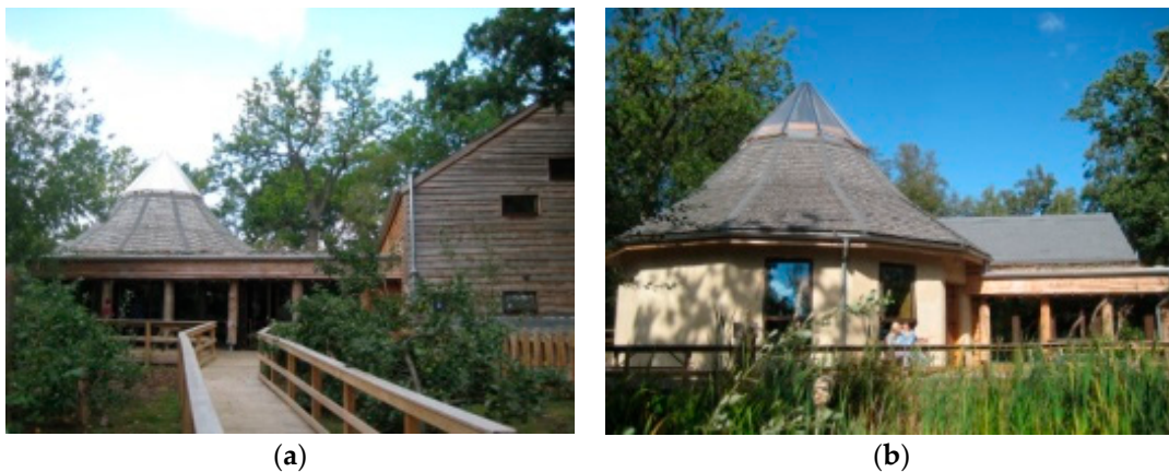
Figure 4. Images of completed building: (a) east-facing elevation; (b) south-facing elevation.
