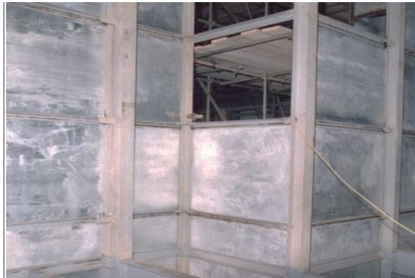
Figure 13. Example of welded panelling and RSJs (© 2016 BAE SYSTEMS. All rights reserved.)
