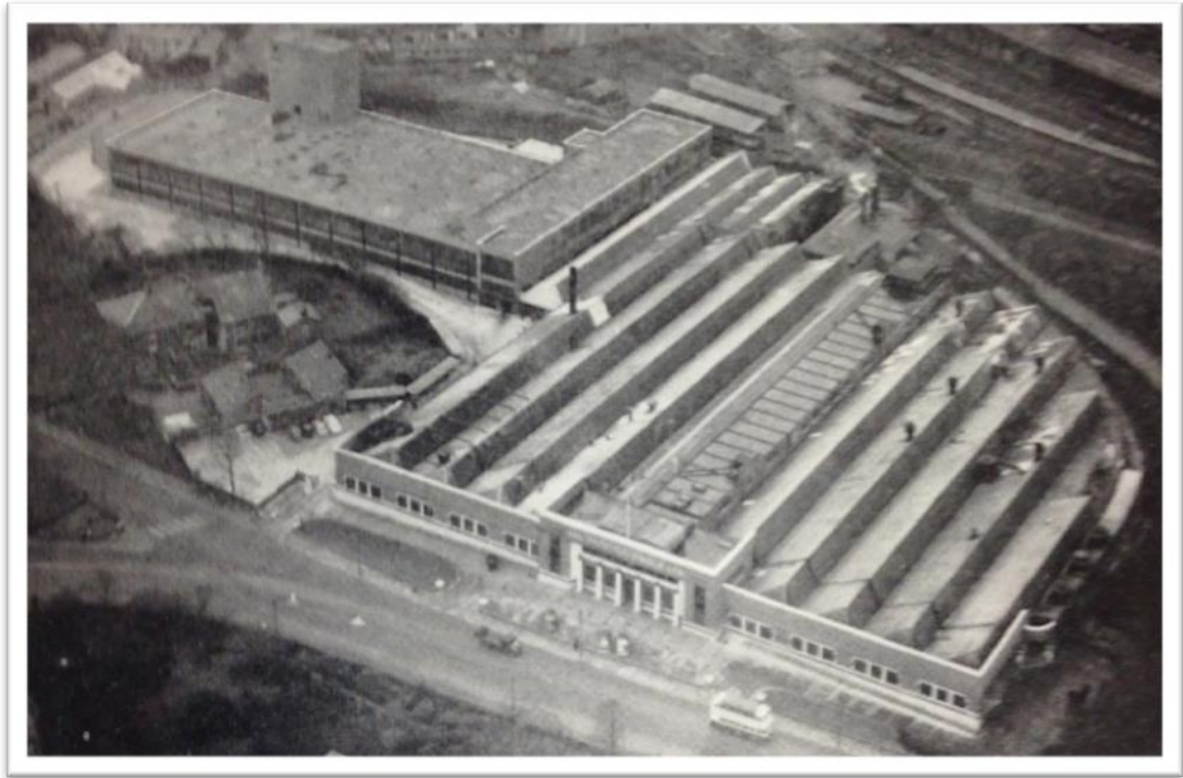
Figure 25: The factory for Platers & Stampers. Source: 'North East Lancashire Industrial Facilities', (Burnley: NELDC, 1956)
