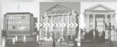
Fig. 7. Re-dressing the building of the Government of Macedonia
