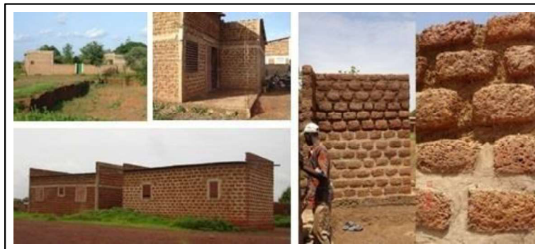
Fig. 2: Typical houses in LDS, either load bearing masonry or with frame concrete.
