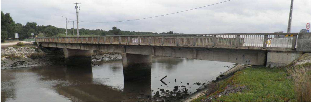
Figure 2: Tercenas bridge lateral view.
