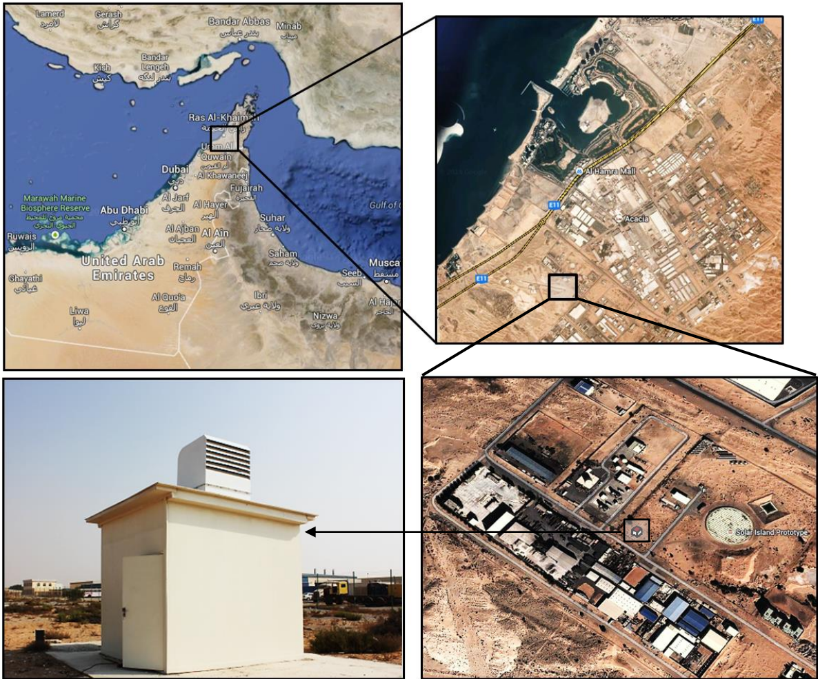
Figure 9 Field test site in Ras Al Khaimah, UAE.
