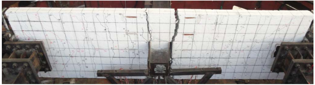
(b)Cracking pattern at top of slab
