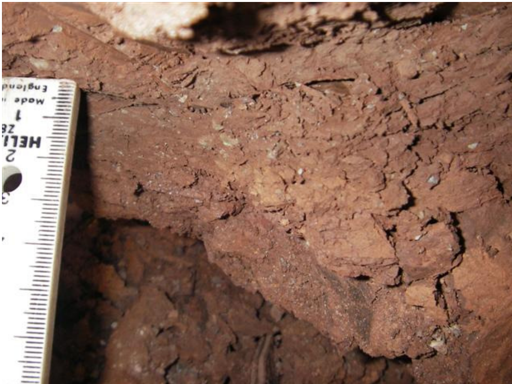
Figure 4.21 The remoulded zone from around pile MR2 at 1000-1457mm below ground level
