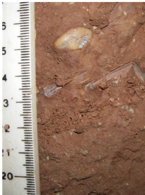
Figure 4.24 The vertical elevation of the remoulded surface of pile MR2 showing free aggregates within the remoulded layers. 1000-1457mm below ground level
