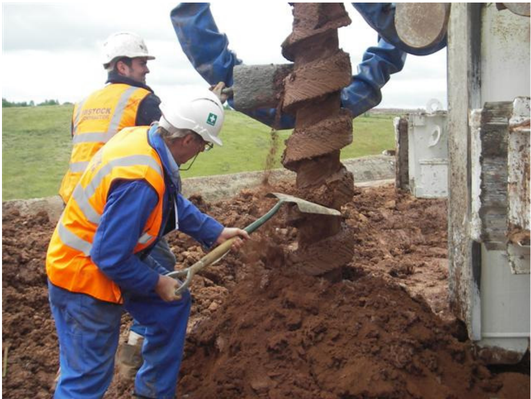
Figure 4.7 The removal of the auger from pile MR3
