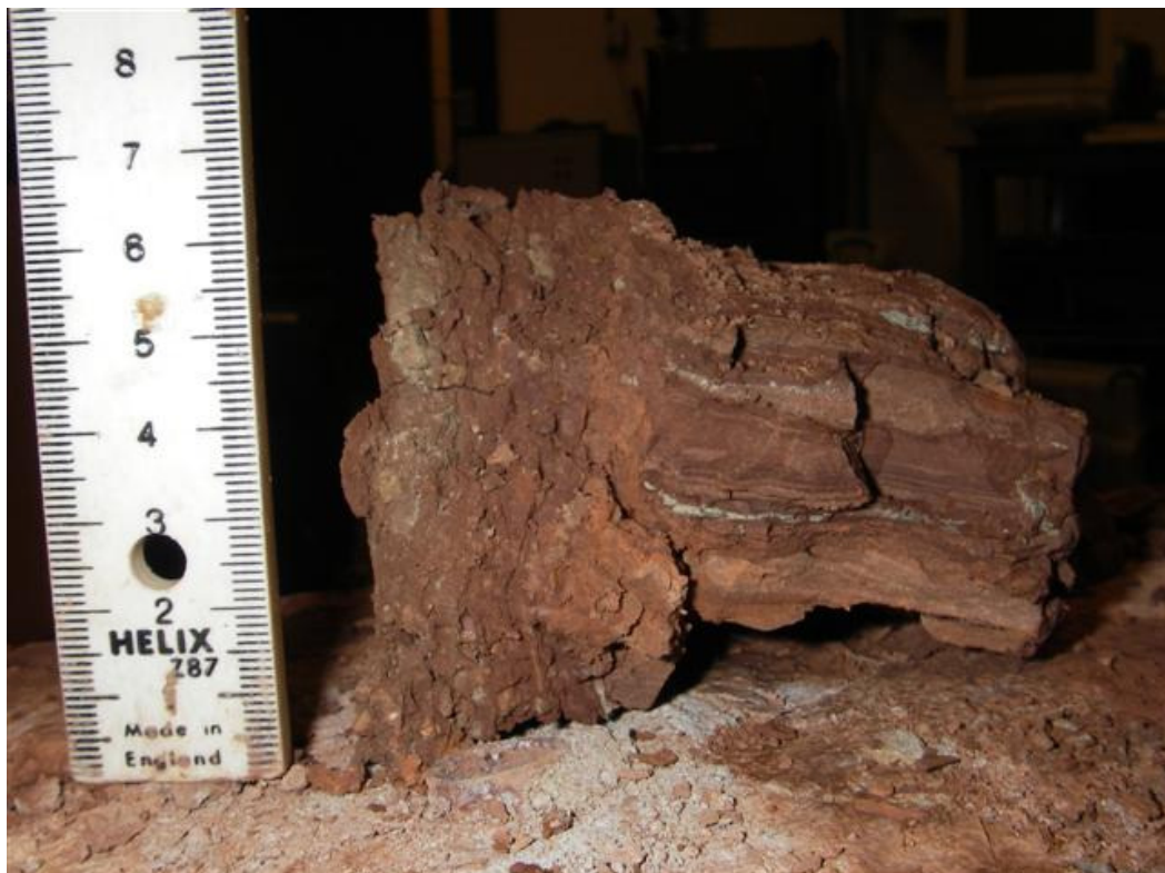
Figure 4.32 Zoning within the remoulded zone of pile MR3 510-860mm below ground level
