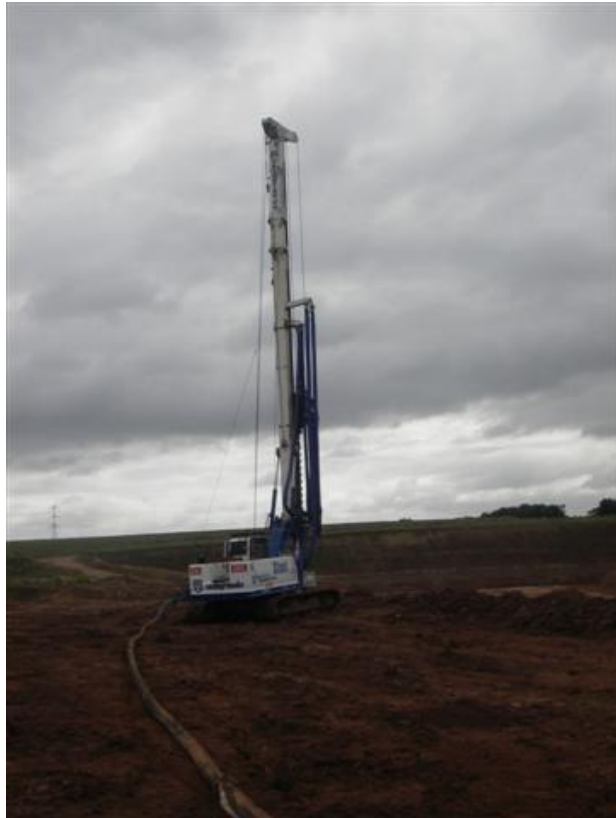
Figure 3.4 The rig used to install test piles
