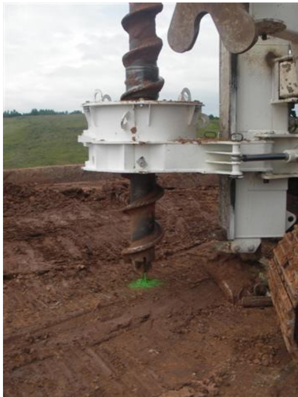
Figure 3.5 The auger used to install test piles
