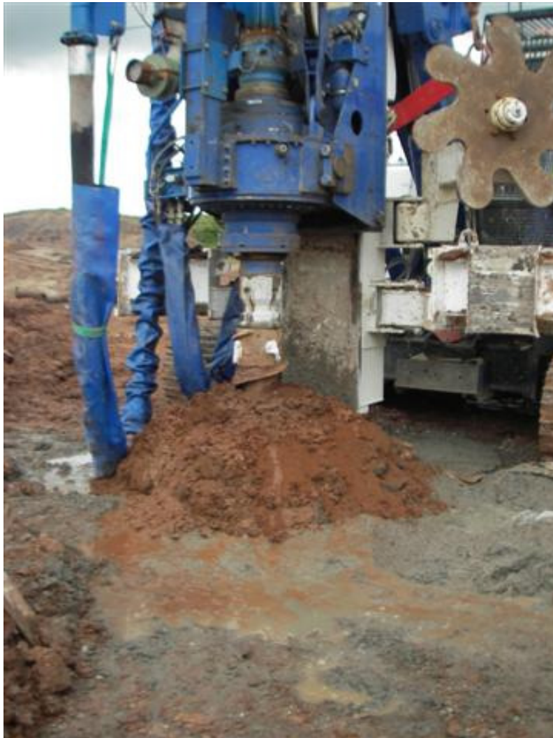
Figure 4.8 The spoil heap produced by the installation of pile MR4
