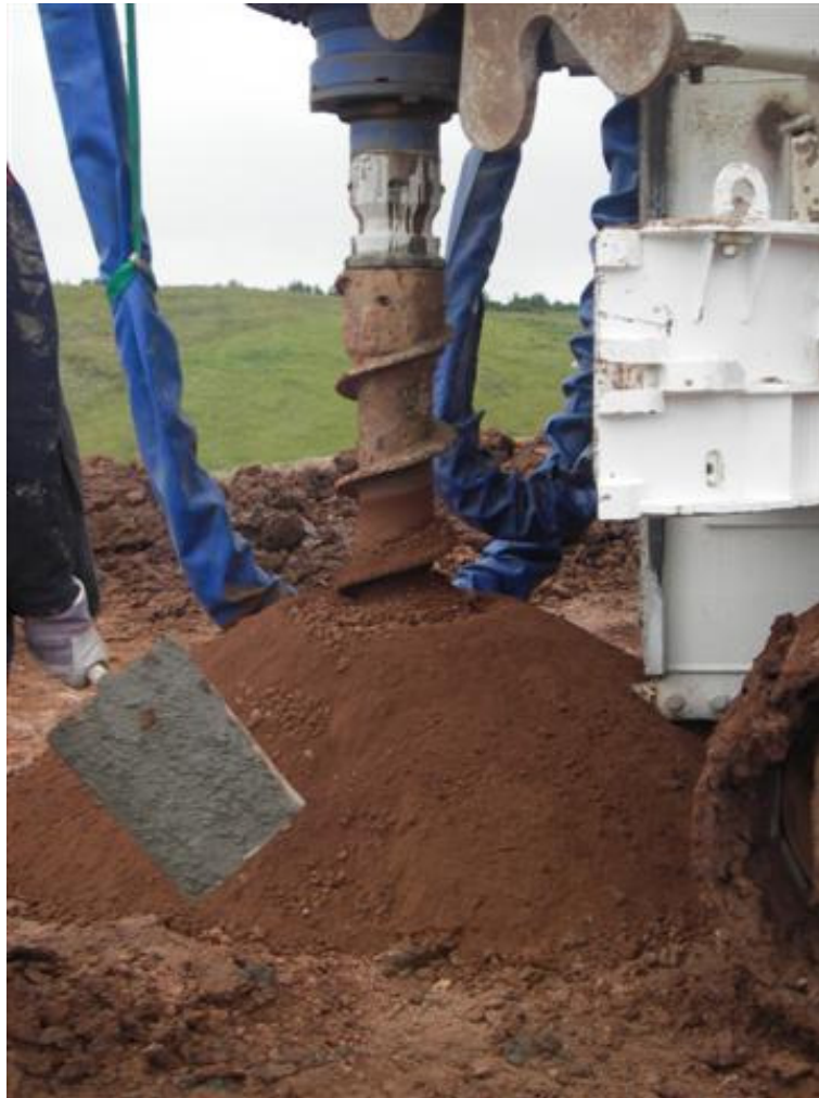
Figure 4.3 The spoil heap for MR1 as the auger was removed.
