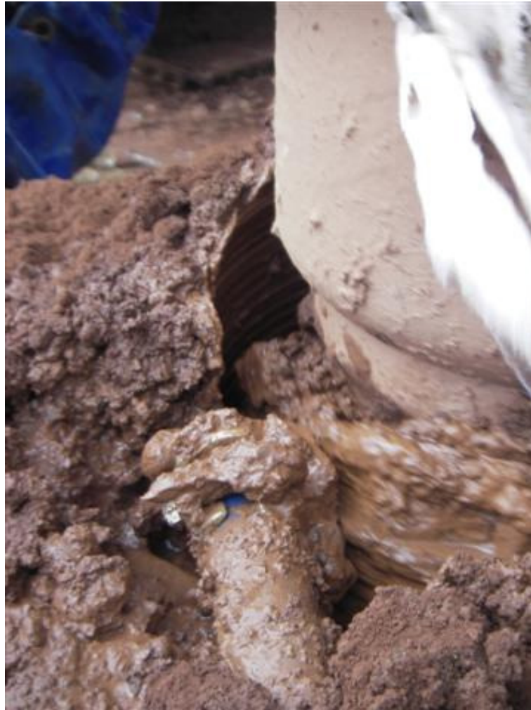
Figure 4.6 The relationship between the auger and the wet soil around pile MR3. Clear markings can be seen on the inner surface of the shaft, along with the hose used to pour water down the shaft
