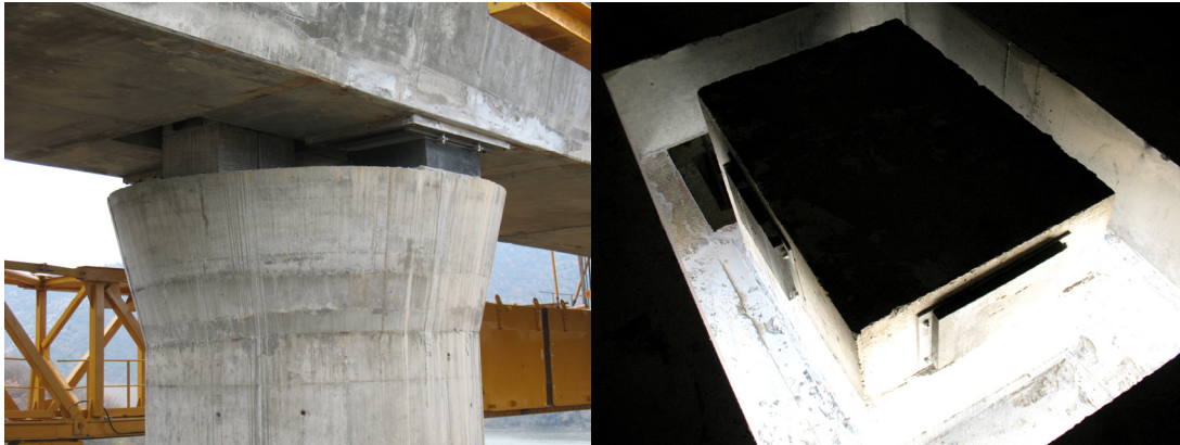
Figure 6: Pier Head and Stopper Details
