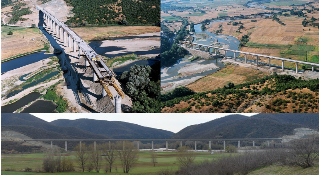
Figure 2: Various aspects of the T12 viaduct
