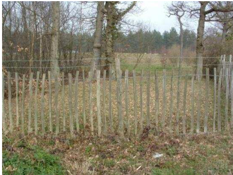
Figure 4.5 Pale fencing, with a top wire
