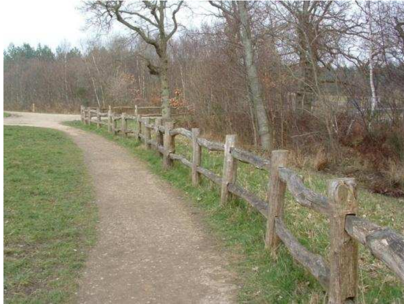
Figure 4.4 Post and rail fencing
