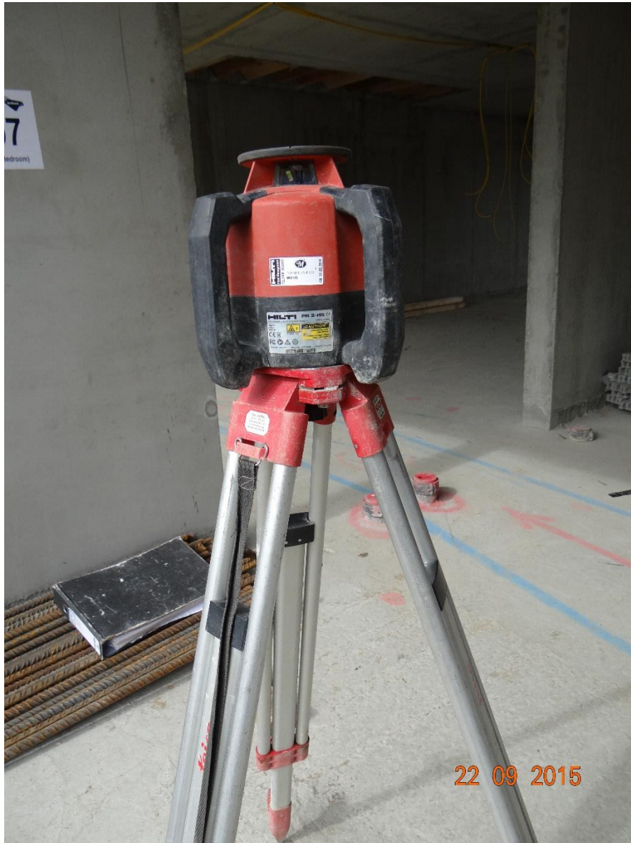
Figure 3.3 Level Observing Deflection on Slab
