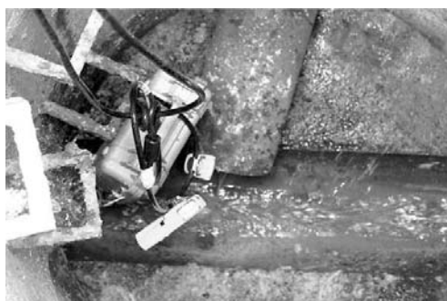
Fig. 1 Equipment setup in a sewer manhole chamber
