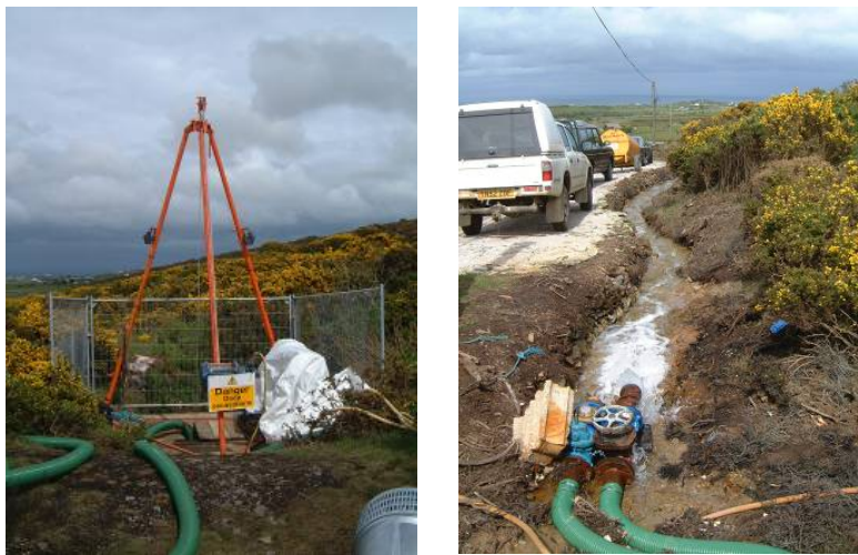
Figure 4. Pumping operations at Gardd Daniel Shaft in 2003.
