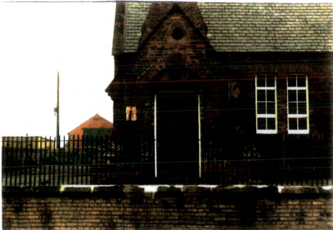
(23) In recent years Bishop Auckland has been the site of quite serious public disorder. This is rumoured locally to be a result of local gang fights. There is much written evidence of such gangs on buildings in Bishop Auckland. For example, the 'Low Life' legends
