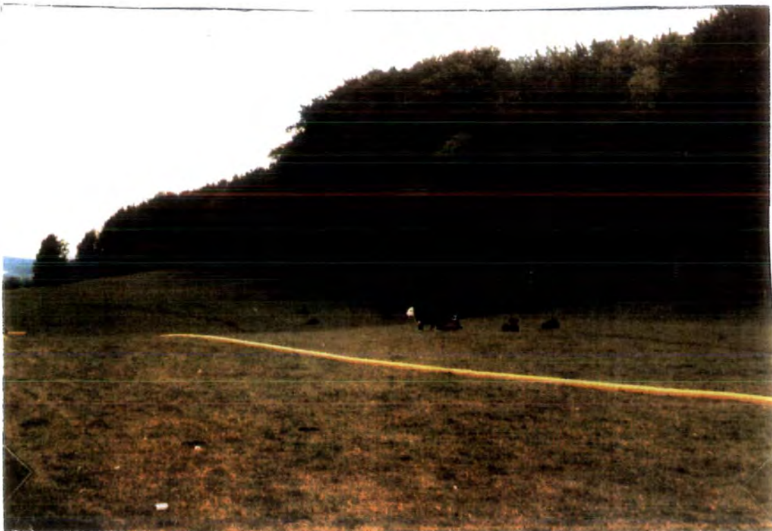
(31) It is not easy to say whether the Wear Valley is rural or urban. In Stanhope and its immediate environs, the local people want the benefits of urbanisation and industrialisation. The yellow plastic pipe will when concealed underground carry mains gas to this area for the first time
